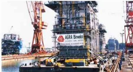
→ 4 Modules Pyrolysis Furnace
