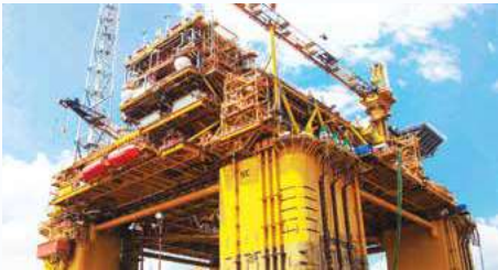
→ Gumusut-Kakap Semi-Submersible Floating Production System (FPS)
