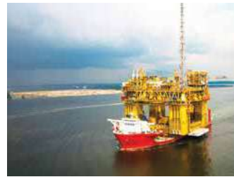
→ Gumusut-Kakap Semi-Submersible Floating Production System (FPS)
