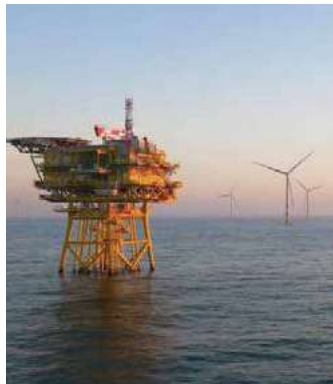
→ Utilising MHB's core competence in offshore fabrication for the offshore wind industry
